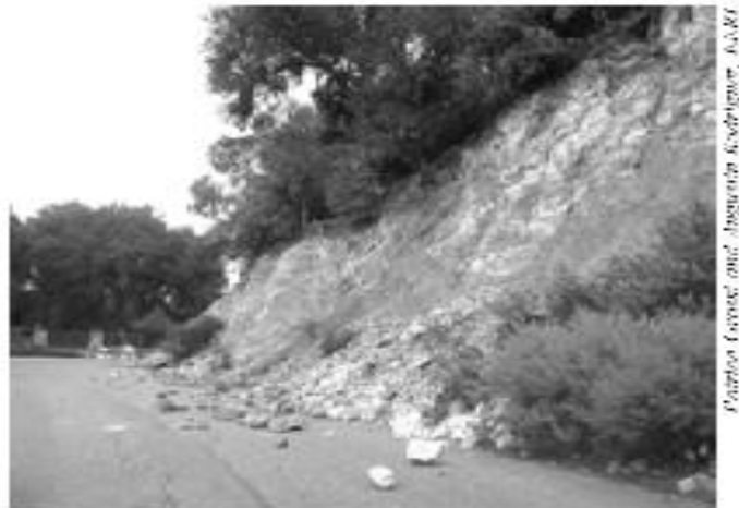
Figure 37 - Landslide. San Simeon Earthquake, December 22, 2003 Landslides on San Gregorio Road in Atascadero, California, only a short distance away from where the homes with the most damage were located.
