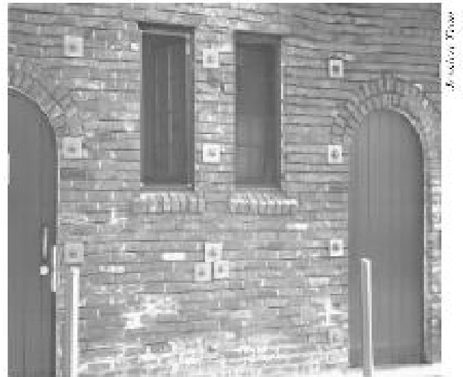
Figure 28 - Bolting of unreinforced masonry wall to steel frame on the inside.
