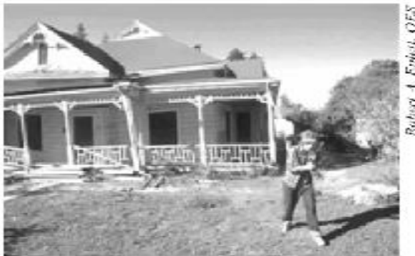
Figure 2 - Loma Prieta Earthquake, Oct. 17, 1989 Home moved off of its foundation and was considered a total loss.
