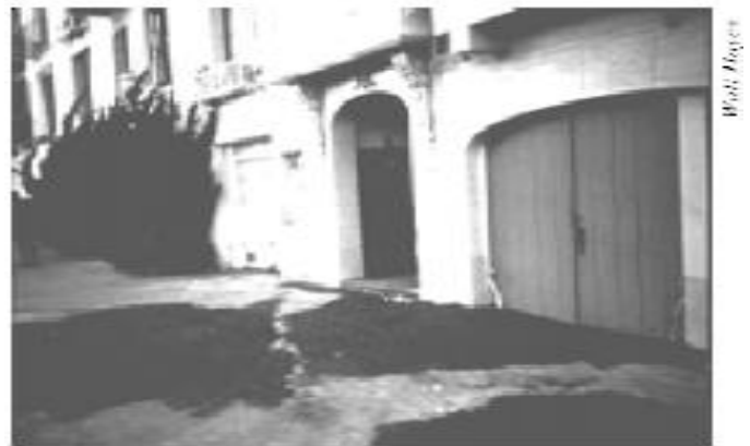
Figure 40 - Loma Prieta Earthquake, October 17, 1989. Lateral spreading, liquefaction and sand boils caused extensive damage in the Marina District of San Francisco, about 60 miles away from the epicenter.
