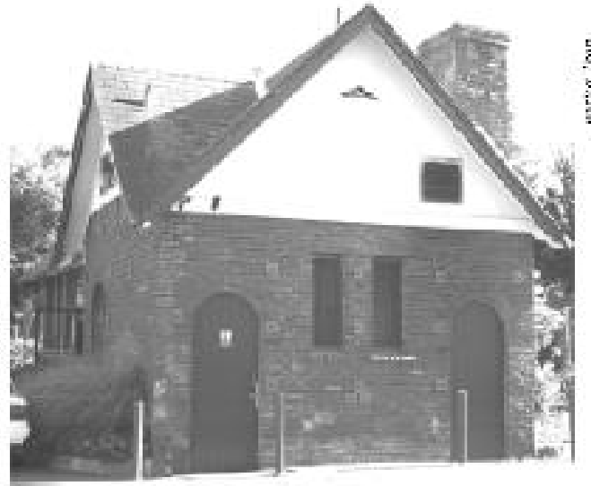
Figure 27 - Unreinforced masonry wall strengthened by installing a steel frame inside.
